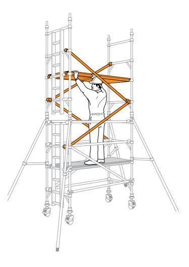
Climb up the inside of the tower and from the protected position of the trapdoor, fit guardrails to the 7th and 8th rungs (in that order) on both sides of the tower.
